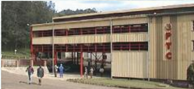
Factory Expansion – Phase II
