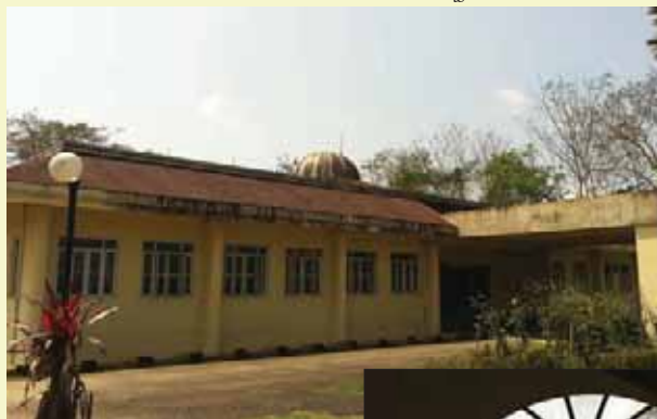
The Main Office with its Glass Dome
